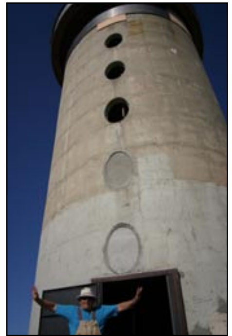
Henry Corning stands in front of the nearly completed bat house.
